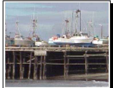
Port Orford Dock Soon to be Replaced
